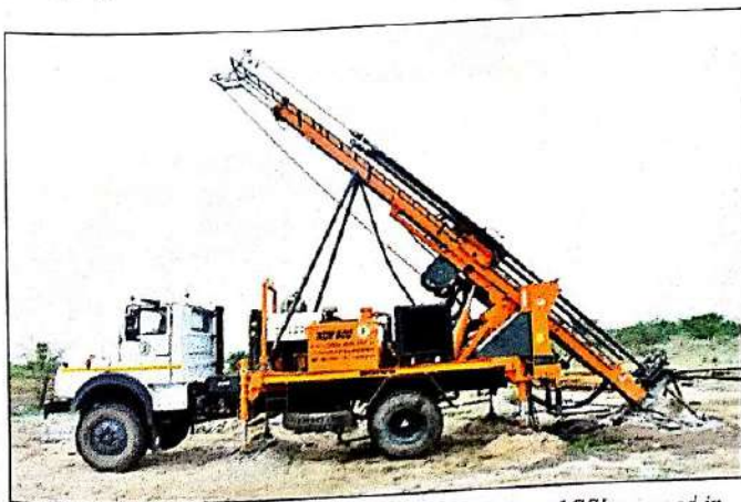
Image 3. Truck mounted hydrostatic drill machine of GSI engaged in mineral exploration work
